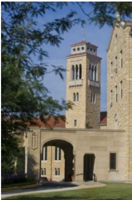
The Canopy Entrance at Assisi Heights
